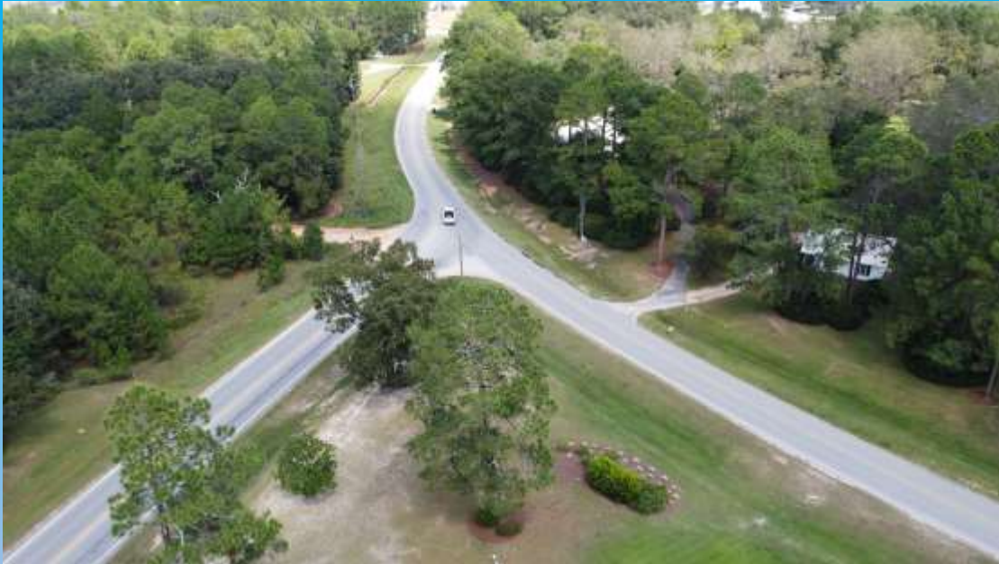
Preconstruction Photo Summer 2023
