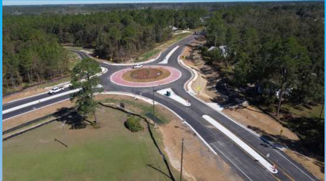
Progress Photo October 2024
