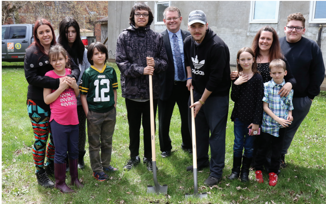
BREAKING GROUND: Families and Habitat for Humanity staff break ground at the soon to be built Leith Street home.
