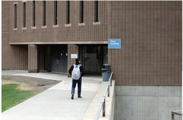
DECADES LONG ERROR: It was discovered the three men's washrooms in the Ryan Building were mistakenly connected to the storm sewer system.
