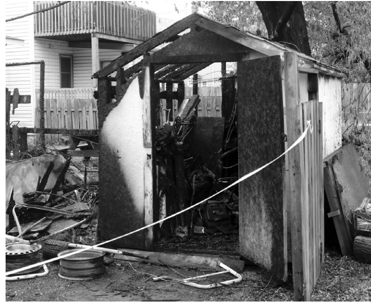
ARSON SUSPECTED: The fire-damaged garage at 325 South Brodie St.
