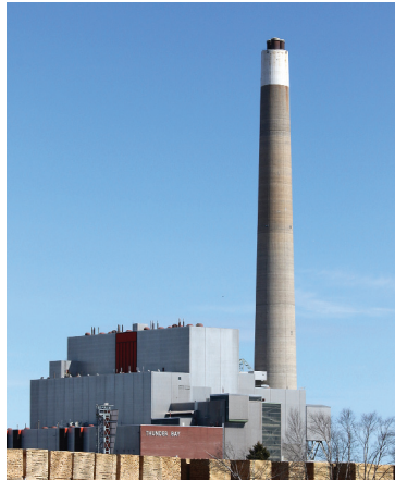
SHUTTING DOWN: Thunder Bay Hydro Power Generating Station.
