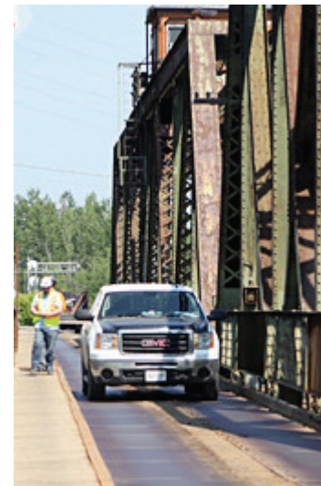
OFF THE HOOK: Courts ruled CN is not bound by a 1906 bridge agreement, which the city will now appeal.
