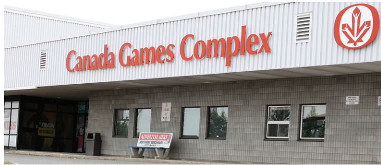
SAFETY CONCERNS: Council voted to award a $1-million contract for Canada Games Complex renovations.
