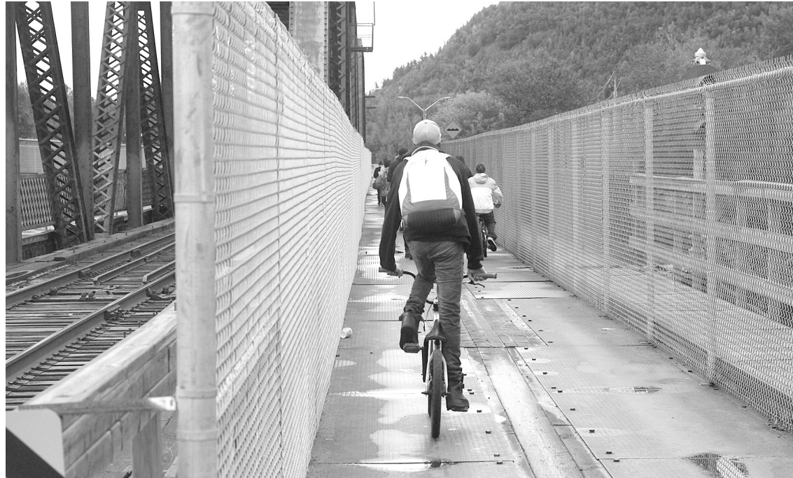
NEARLY FIVE YEARS: Cyclists can still use the James Street Swing Bridge, but motorists have been out of luck since October 2013.
