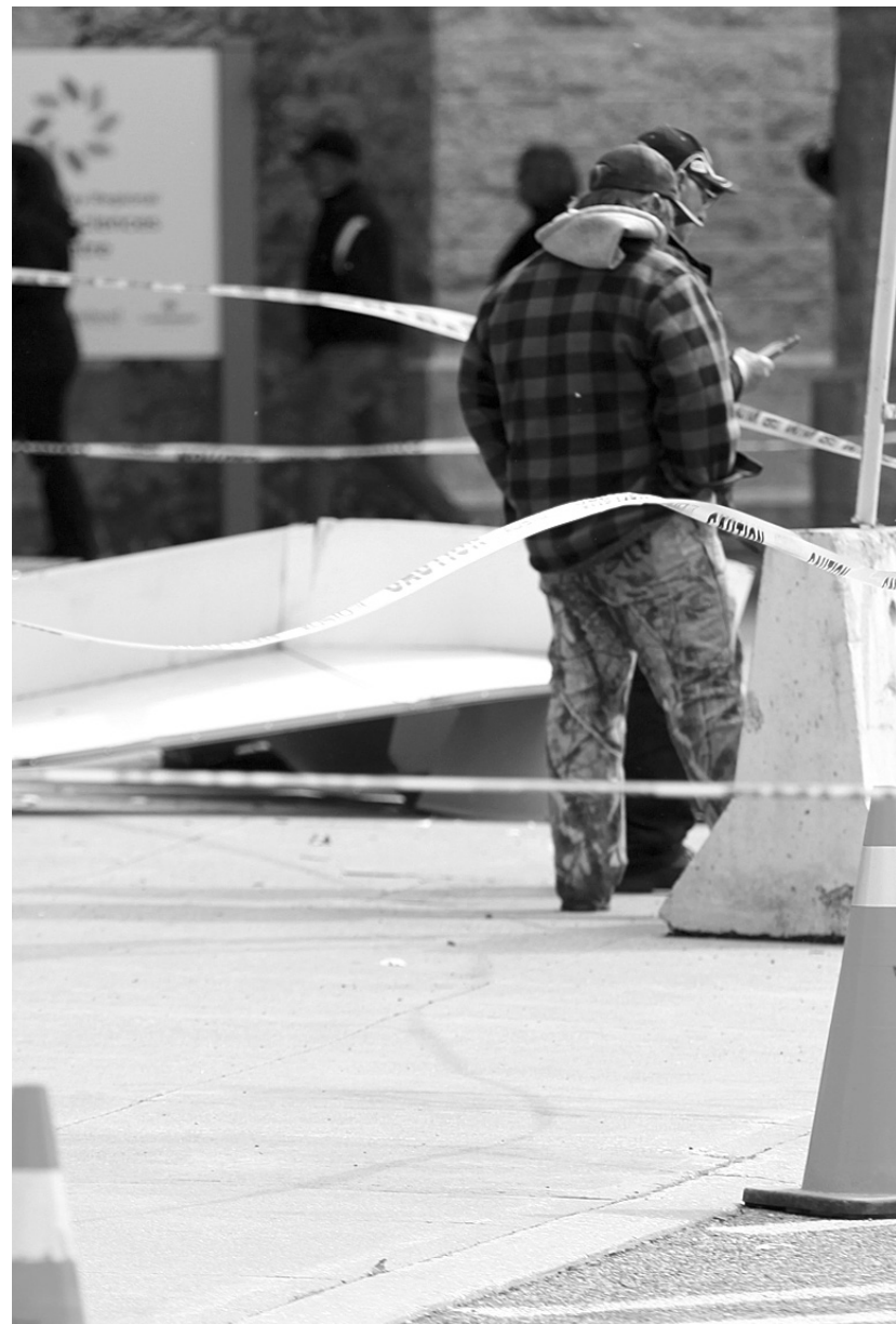
WIND DAMAGE Large pieces of debris are seen outside the main entrance to the Thunder Bay Regional Health Sciences Centre last Friday. No one was injured.
