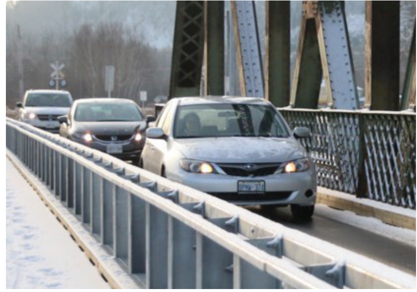
SIX YEAR DELAY: Traffic began traversing the James Street Swing Bridge on Friday night.
