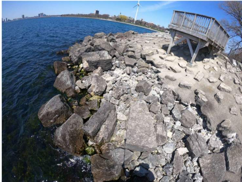
Figure 2.3: Deteriorated grouted armour revetment protection at west headland (Baird 2022-04-29)
