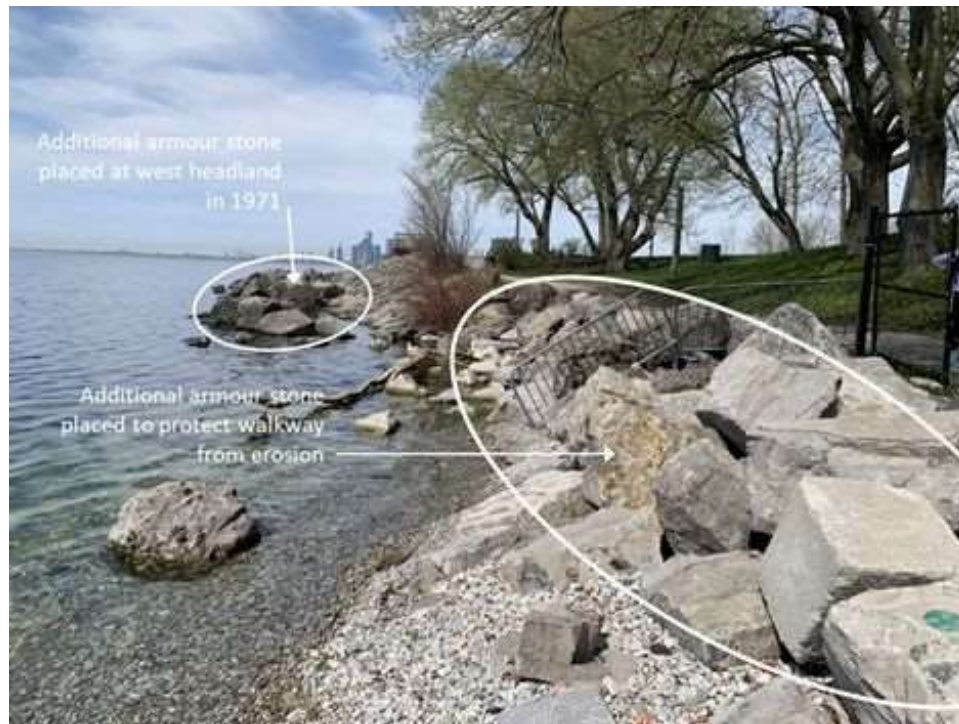
Figure 2.7: Additional armour stone placed at the west headland and at the west end of the beach to provide erosion protection to perimeter of lakefill (Baird 2023-5-06)
