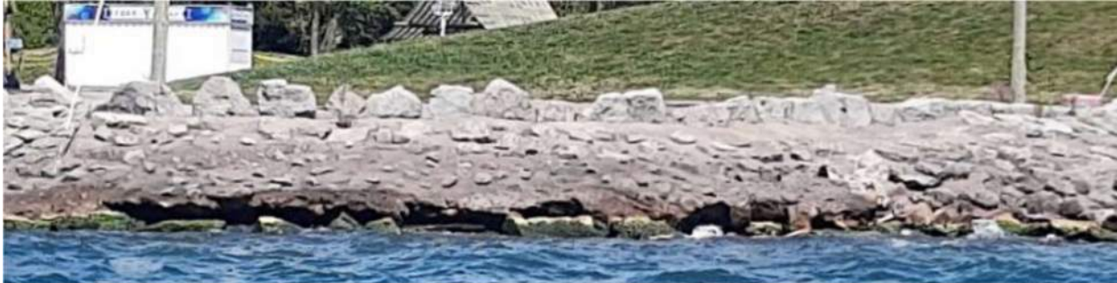
Figure 2.4: Deterioration of grouted stone revetment at east headland (from Jacobs, 2020)
