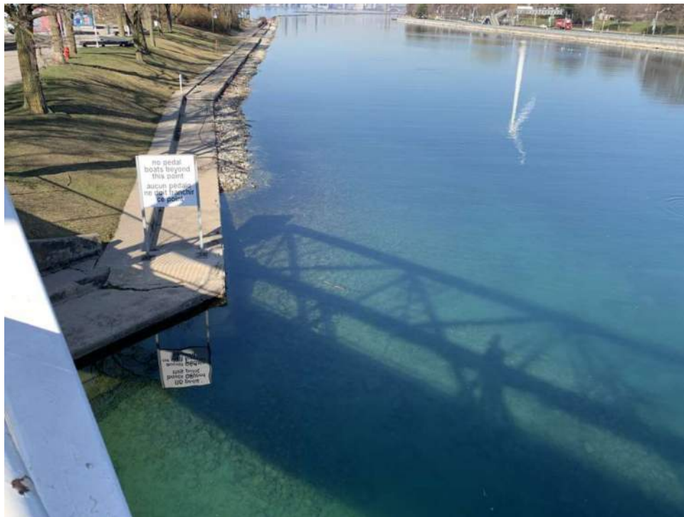
Figure 2.9: View looking west of the north wall of West Island (left-hand side of photo) with rip rap revetment protection.
