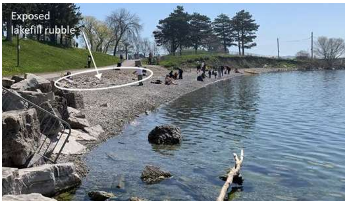
Figure 2.6: South shore with exposed lakefill rubble at the back of the beach (Baird 2023-05-06)
