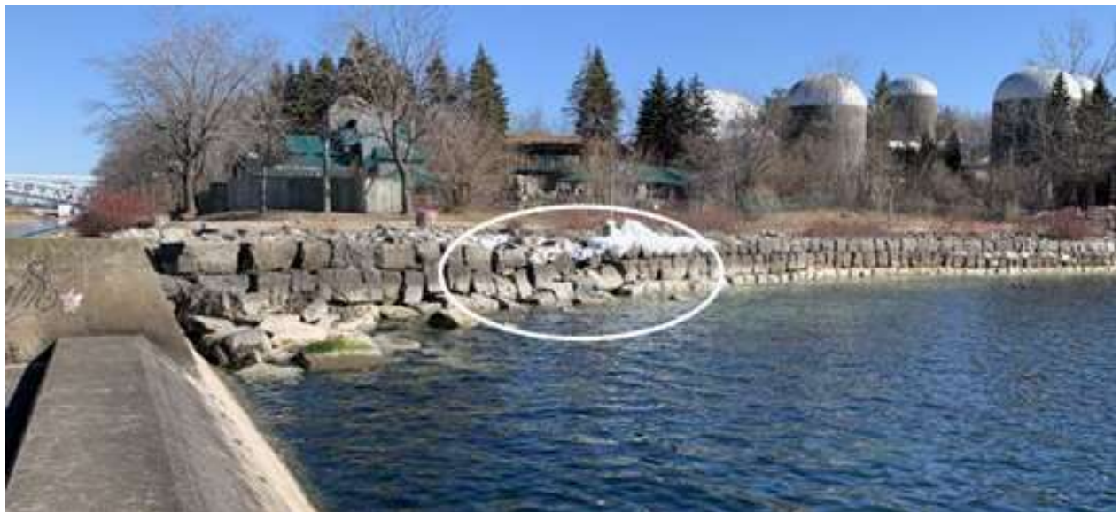
Figure 2.2: Collapsed portion of stacked armour stone seawall at west shore
