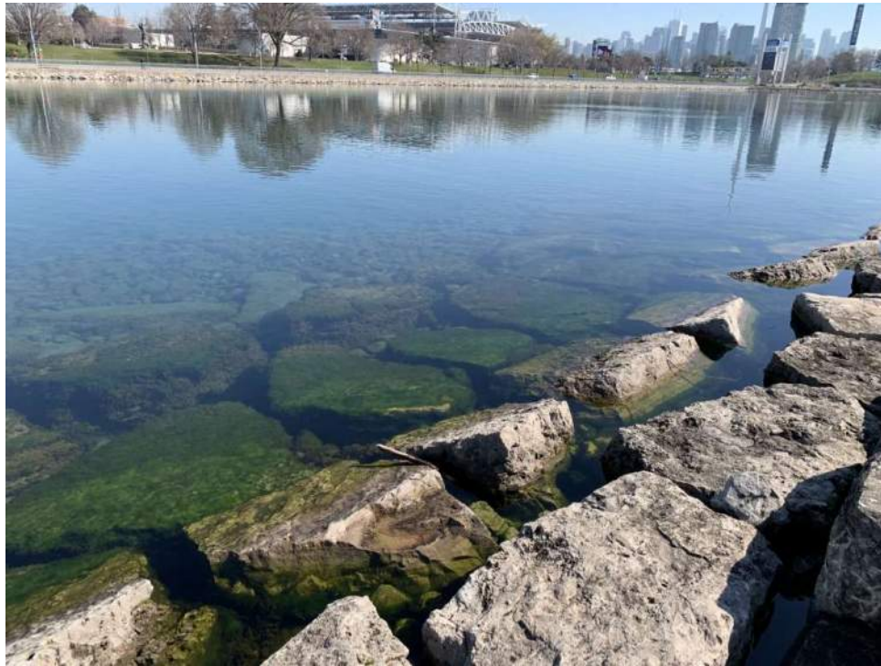
Figure 2.12: Armour stone along the inner side (north side) of the westerly portion of the existing breakwater
