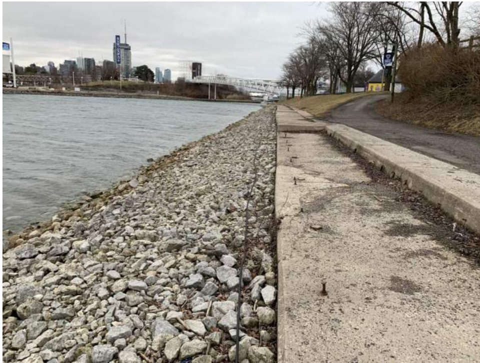
Figure 2.10: Rip rap revetment along the north wall of West Island
