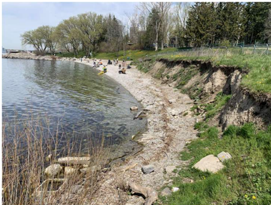
Figure 2.8: Narrow south shore and significant erosion of lakefill perimeter (Baird 2023-05-06)
